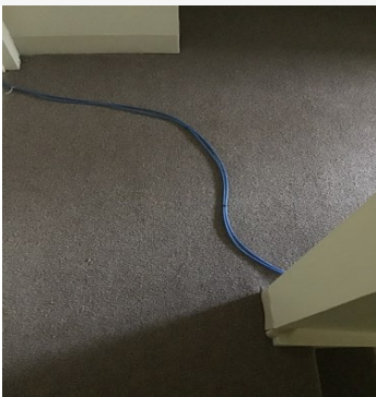
Building 4 Unit 4-21 - Halls/Corridors/Stairs - Floor - Hard - Apr 24 2023 1:58PM - T Knight CAPTION: Cable in floor across hall
