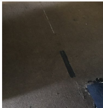
Building 4 Unit 4-21 - Living Room - Floor - Soft - Apr 24 2023 1:52PM - T Knight CAPTION: Carpet pulling at seams ... duck tape in place
