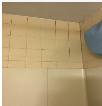
Building 6 Unit 6-28 - Bathroom 1 - Ventilation/Exhaust - Apr 25 2023 9:30AM - T Knight - CAPTION: Caulk needed between tub and wall .... Some mold or mildew also on tile grout
