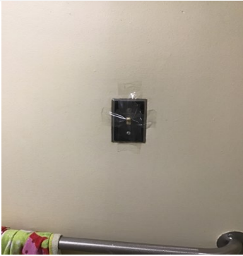
Building 3 Unit 3-15 - Bathroom 1 - Call- for-Aid System - Apr 24 2023 12:45PM - T Knight CAPTION: Cord has been cut in all three ... replace cords
