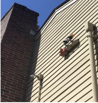
Building 2 - Exterior Wall - Chimney - Apr 25 2023 10:50AM - T Knight CAPTION: Building 2 near Apt 19 chimney deteriorated
