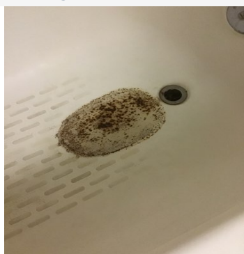
Building 5 Unit 5-27 - Bathroom 1 - Shower/Tub - Hardware - Apr 25 2023 9:14AM - T Knight CAPTION: Tub is rusting .... Shower wall starting to crack
