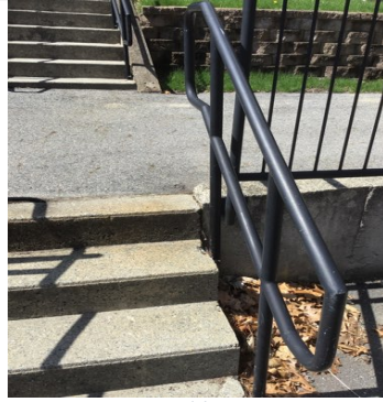
Site - Walkway/Steps - Handrail - Apr 25 2023 11:02AM - T Knight CAPTION: Hand rail is loose front of unit 12
