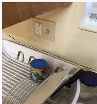
Building 2 Unit 2-08 - Kitchen - Wall Covering and Finish - Interior - Apr 24 2023 10:47AM - T Knight CAPTION: Repair crack in wall behind sink
