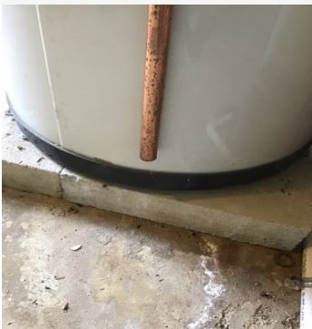
Building 6 - Local Systems - Pipes/drains - Apr 25 2023 10:30AM - T Knight CAPTION: Water heater and other extension pipes must be no higher than 6 inches or lower than two inches from floor for nspire
