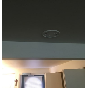
Building E Unit E2-37 - Living Room - Smoke Alarms - Aug 31 2023 3:22PM - T Knight CAPTION: Living room smoke detector missing
