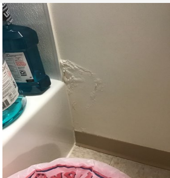
Building B Unit B1-9 - Bathroom 1 - Wall Covering and Finish – Interior - Aug 14 2023 10:14AM - T Knight CAPTION: Wall Water damage between tub and sink
