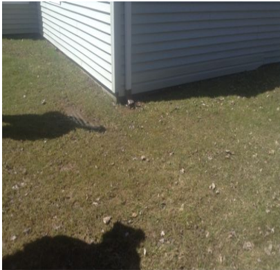
26 Community Building Roofing - Downspout/Gutter
