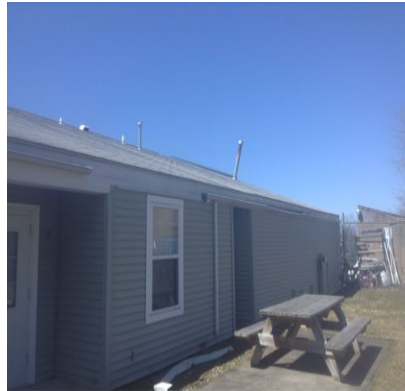
27 Community Building Roofing - Downspout/Gutter
