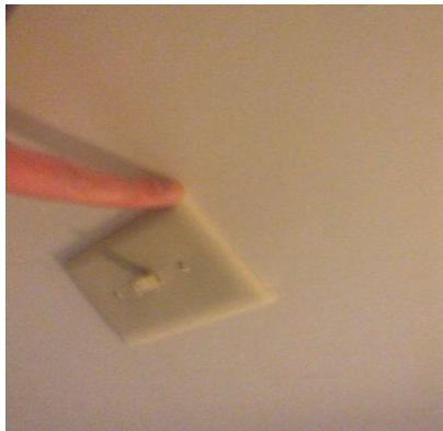
50 05-A Unit 02 Bedroom 1 - Outlets/Switches
