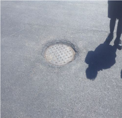
7 Site Roads/Parking/Curbs - Roads/Parking/Curbs
