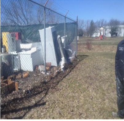
1 Site Fence/Gate - Fence - Security/Safety
