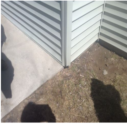
23 Community Building Exterior Walls - Walls
