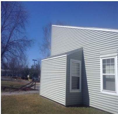
29 Community Building Roofing - Soffit/Fascia
