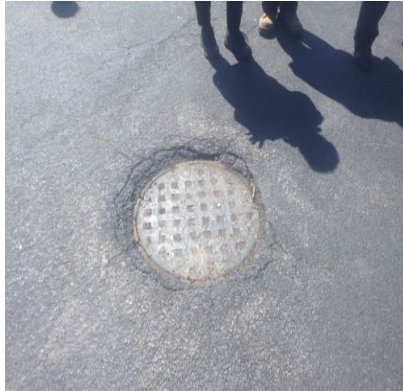
8 Site Roads/Parking/Curbs - Roads/Parking/Curbs
