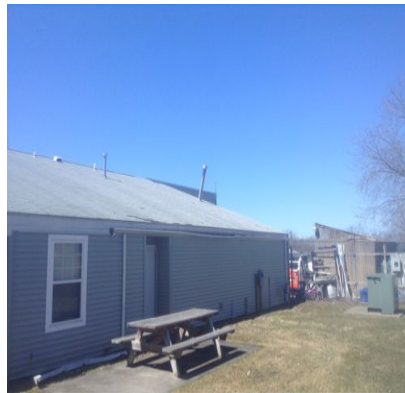
30 Community Building Roofing - Vents
