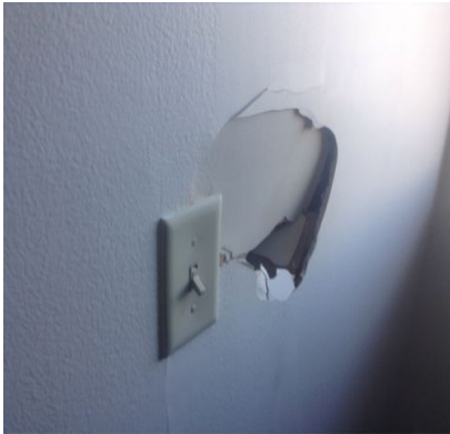
58 05-A Unit 03 Halls/Corridors/Stairs - Walls
