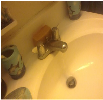
44 05-A Unit 01 Bathroom 1 - Sink
