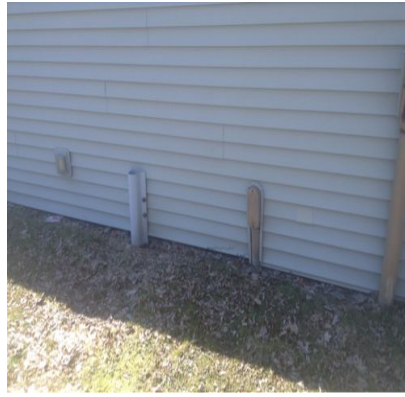
24 Community Building Exterior Walls - Walls
