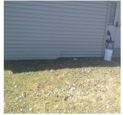
25 Community Building Exterior Walls - Walls
