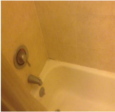
43 05-A Unit 01 Bathroom 1 - Shower/Tub - Stall
