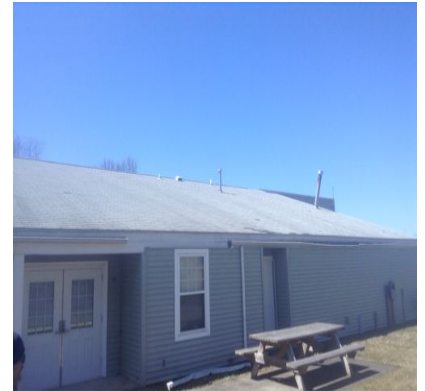
28 Community Building Roofing - Roof Surface/Shingle
