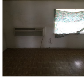
16 608 Unit 608-17 General Unit - General Unit
