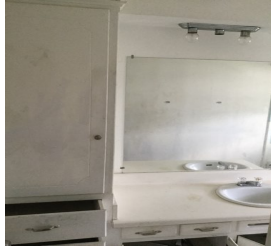
18 608 Unit 608-17 General Unit - General Unit
