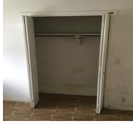
19 608 Unit 608-17 General Unit - General Unit
