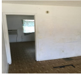
15 608 Unit 608-17 General Unit - General Unit
