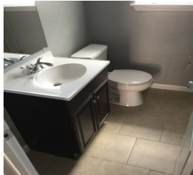
26 612 Unit 612-24 Bathroom 1 - Sink Faucet
