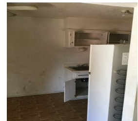
13 608 Unit 608-17 General Unit - General Unit
