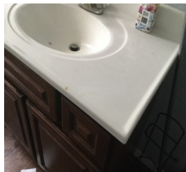
11 608 Unit 608-11 Bathroom 1 - Countertop
